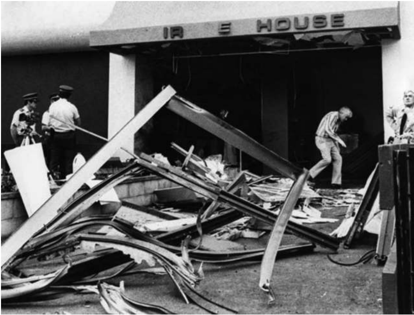
Figure 10.1: The broken front of the Wanganui Computer Centre in 1982 after the bombing.
